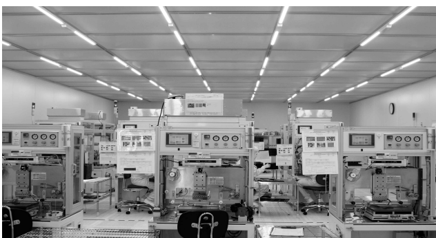
Fig. 10. Installation of TD LED Lighting Fixture(1)
